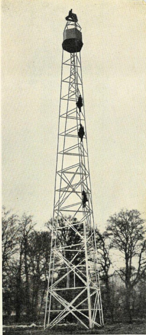
One of the towers erected for triangulation when there are no hills or mountains about.
