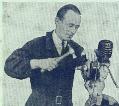
Removing flywheel with special "hammer tight" spanner
